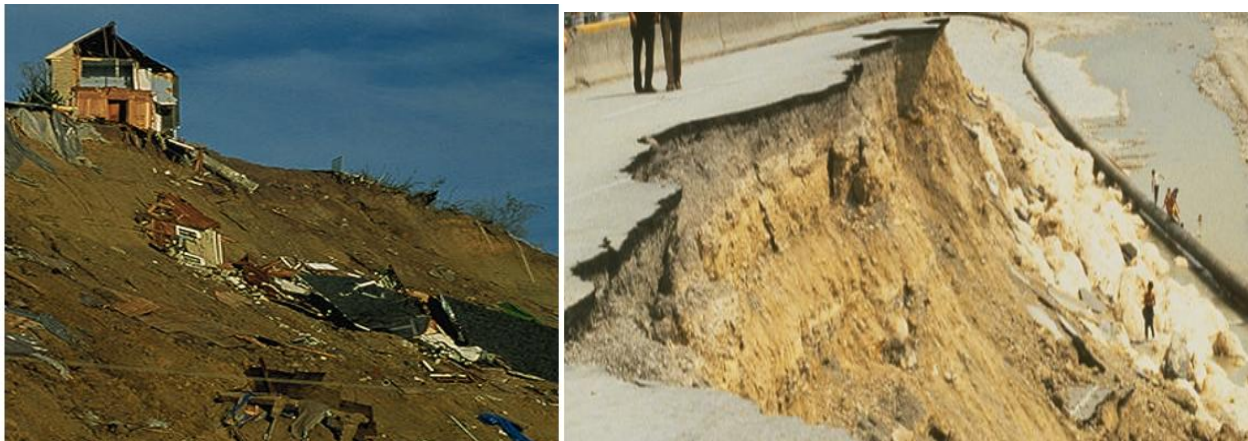
Figure 9: the effect of Earth subsidence on damaged of road and building
